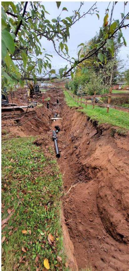
Picture from our current construction project as Jake's Excavating replace water lines in the city
